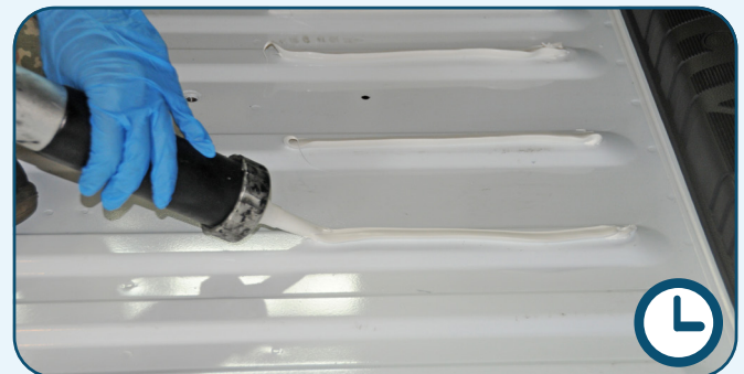
Glue with caulking gun
